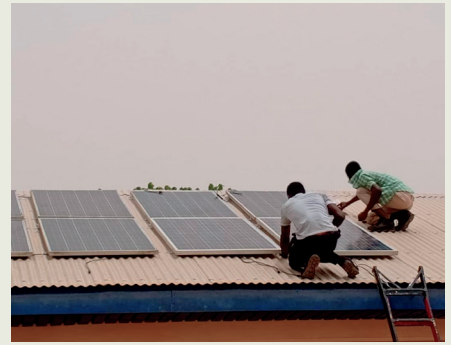
Workers install solar panels at the Sisters of Mary Immaculate convent in Damongo, Ghana, bringing sustainable energy to the community.
